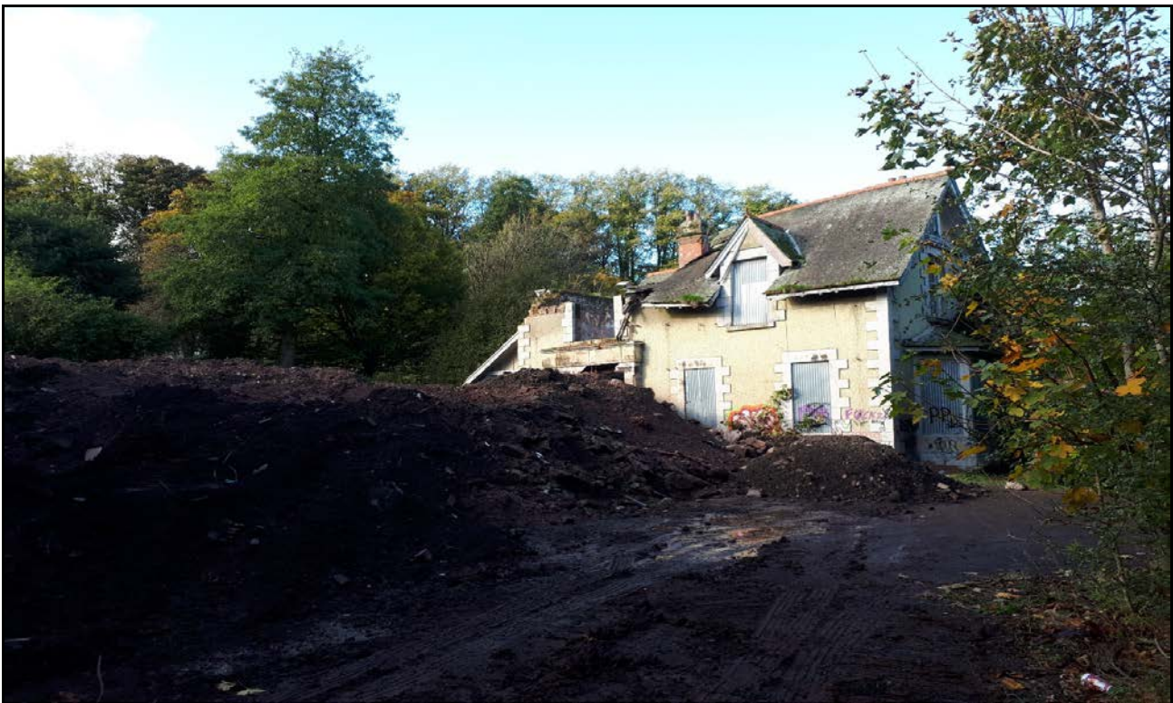
Annexe building – photograph taken October 2021
