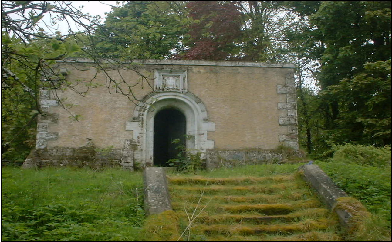
Water Tower – photograph taken 2019
